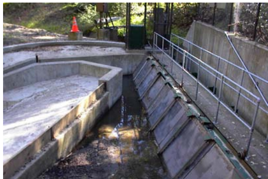
Inclined Flat Plate Screen
