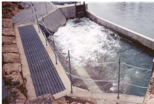
Screen with Air Burst Operation
