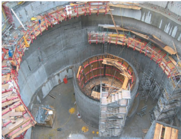
Shaft Casting and Backfilling
