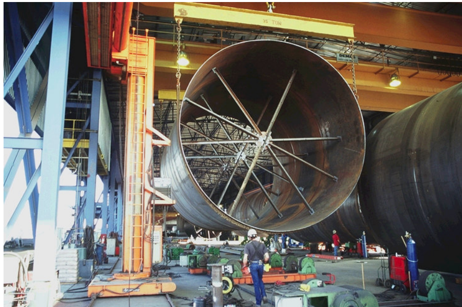
Figure 2: Fabrication of 21-Foot-Diameter Steel Pipe by Schuff Steel Company
