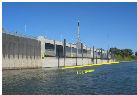
RD 108 On-Bank Intake
