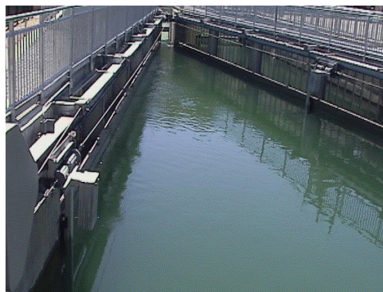
Chevron Intake in Service
