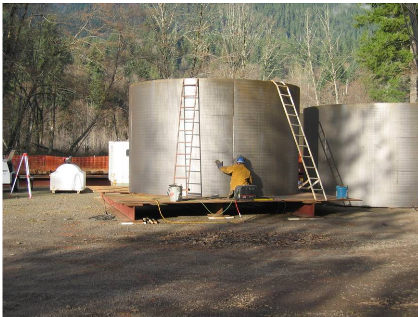
Figure 3: On-Site Fabrication of Bent Plate Steel Pipe
