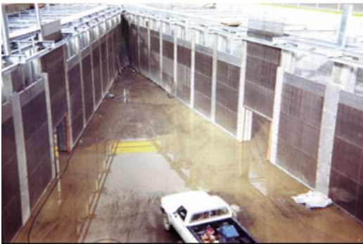
Chevron Screen (Dry)
