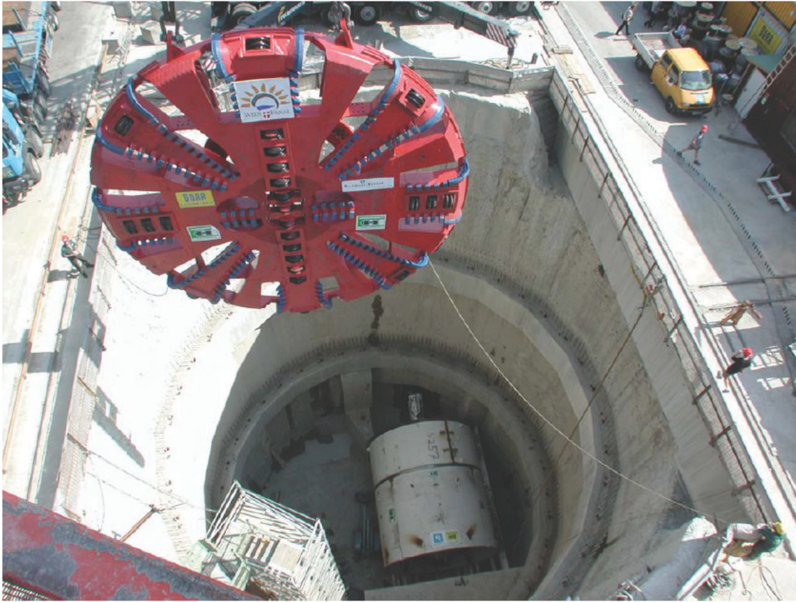
TBM Assembly in the Launching Shaft
