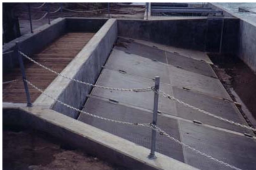
Inclined Flat Plate Screen
