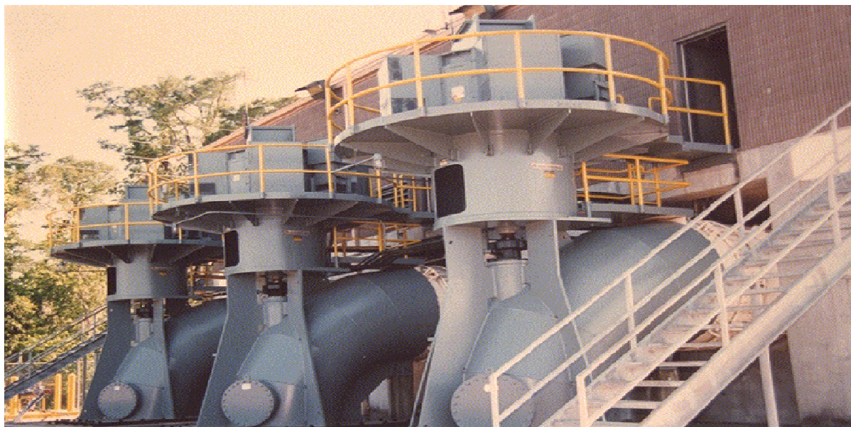
Figure 3: Vertical Column Mixed Flow Pumps
