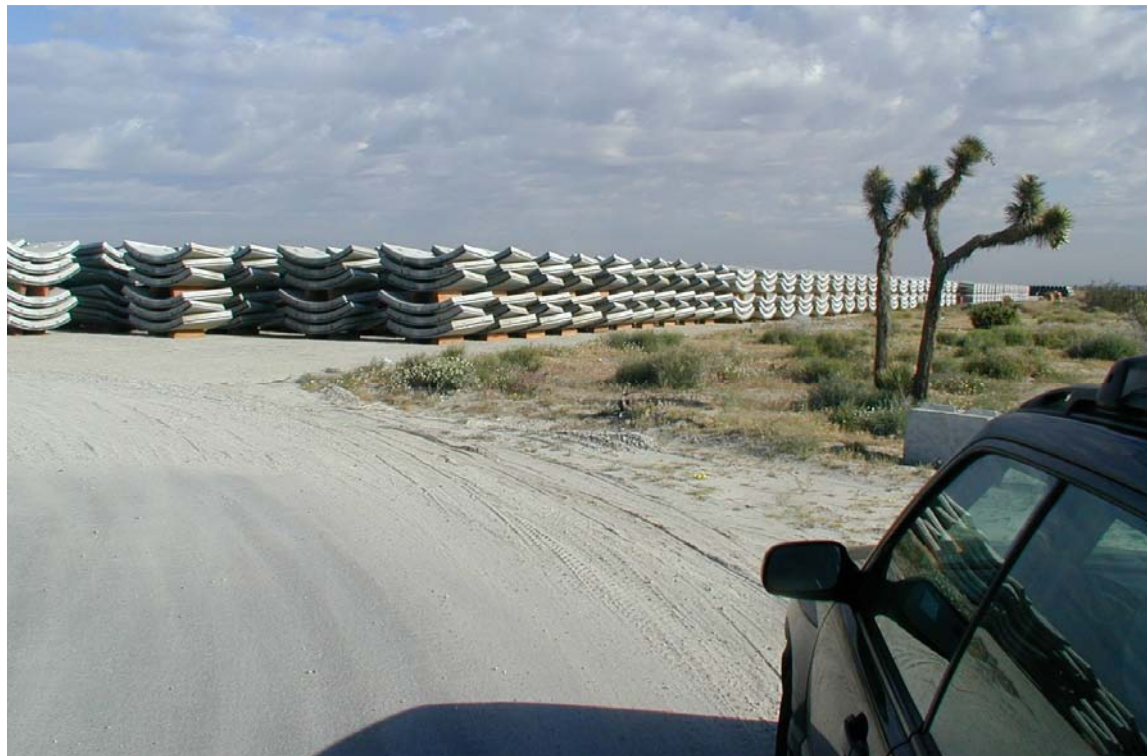
Typical Casting Yard
