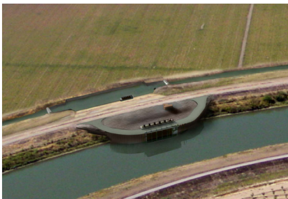
Sutter Mutual On-Bank Intake
